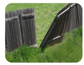
**Before:** The Posts are rotted and have weakened to the point of where the fence has now started to lean. No worries, call The Post Doctor.
